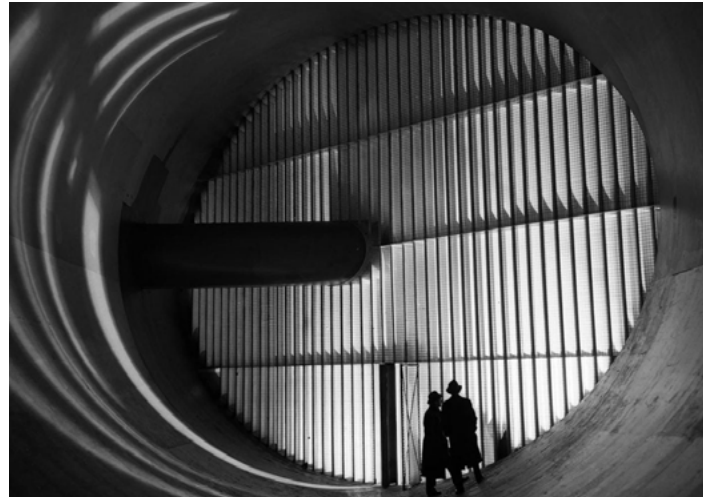
Turning vanes inside the Altitude Wind Tunnel. Credit: NASA.
