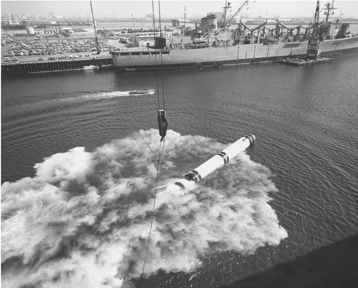
Figure No. E-5. Solid rocket booster drop tests at the Long Beach Naval Shipyard, California, 1973.
