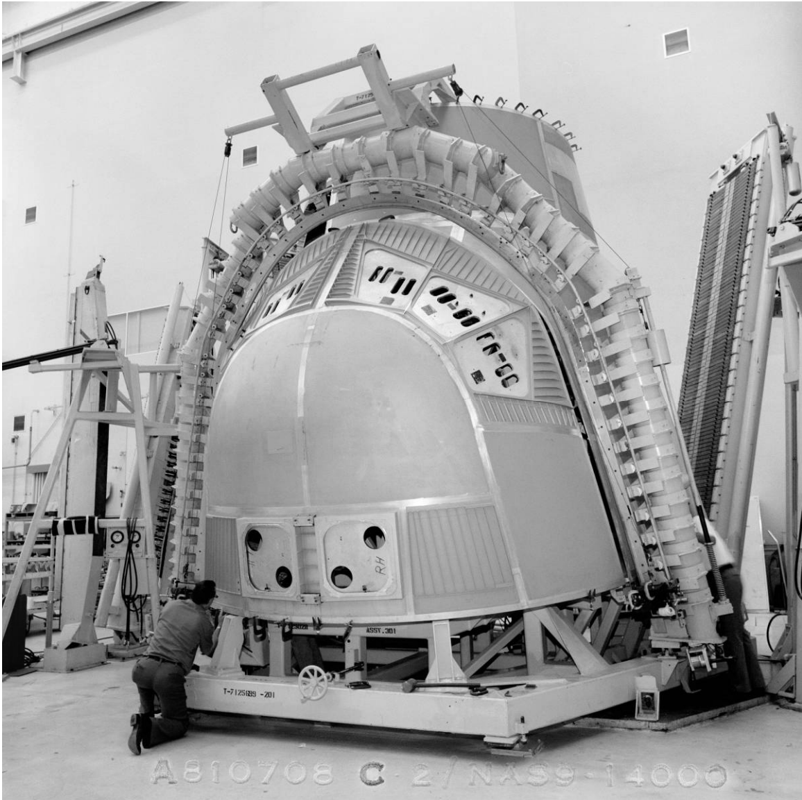
Figure B-8. Primary structure assembly for Discovery's crew module in weld tool, NAR Building 290, Downey, California, July 8, 1981. Source: NASA, Johnson Space Center Image Repository, JSC2010-03119.
