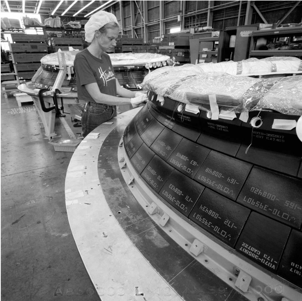
Figure B-55. Installation of HRSI on one of Discovery 's SSME dome heat shields at AFP 42, August 9, 1983.
