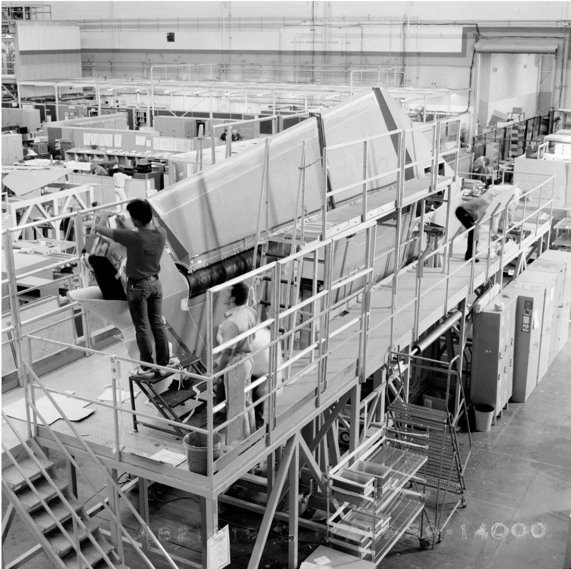
Figure B-30. Installation of TPS on Discovery's vertical stabilizer, AFP 42, October 19, 1982. Source: NASA, Johnson Space Center Image Repository, JSC2010-03353.
