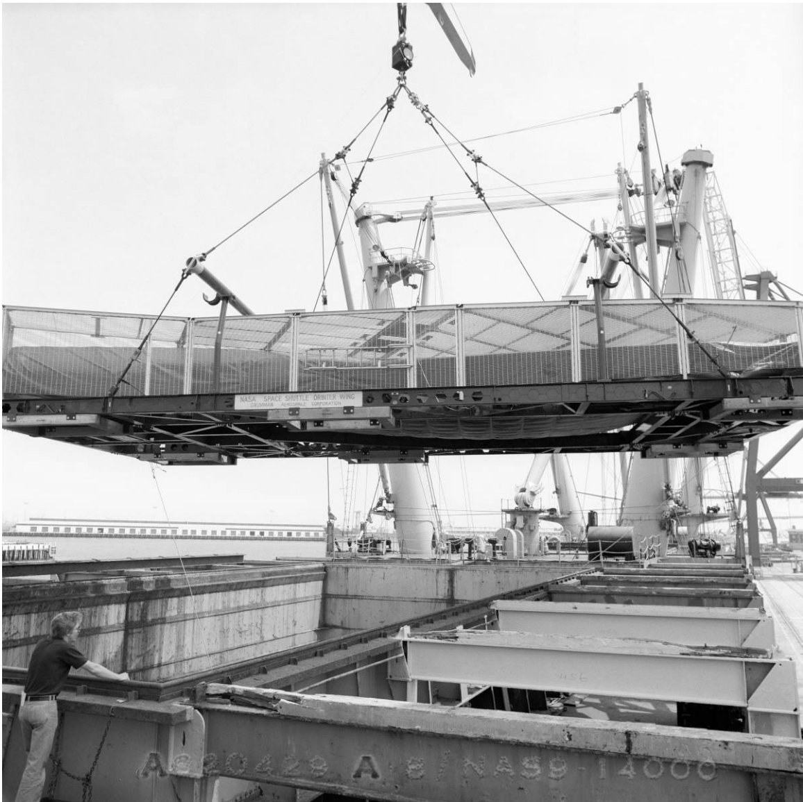
Figure B-21. Discovery's port wing being offloaded from ship at the Los Angeles Harbor for delivery to AFP 42, April 29, 1982.
