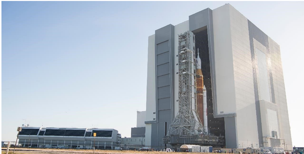
Figure 3-4. Exploration Ground Systems
