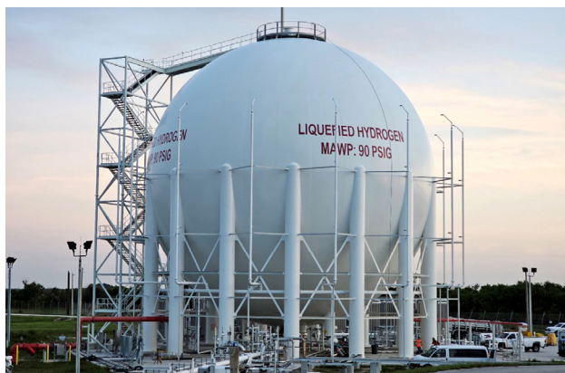
Figure 1: The new 1.3-million-gallon LH 2 tank.
