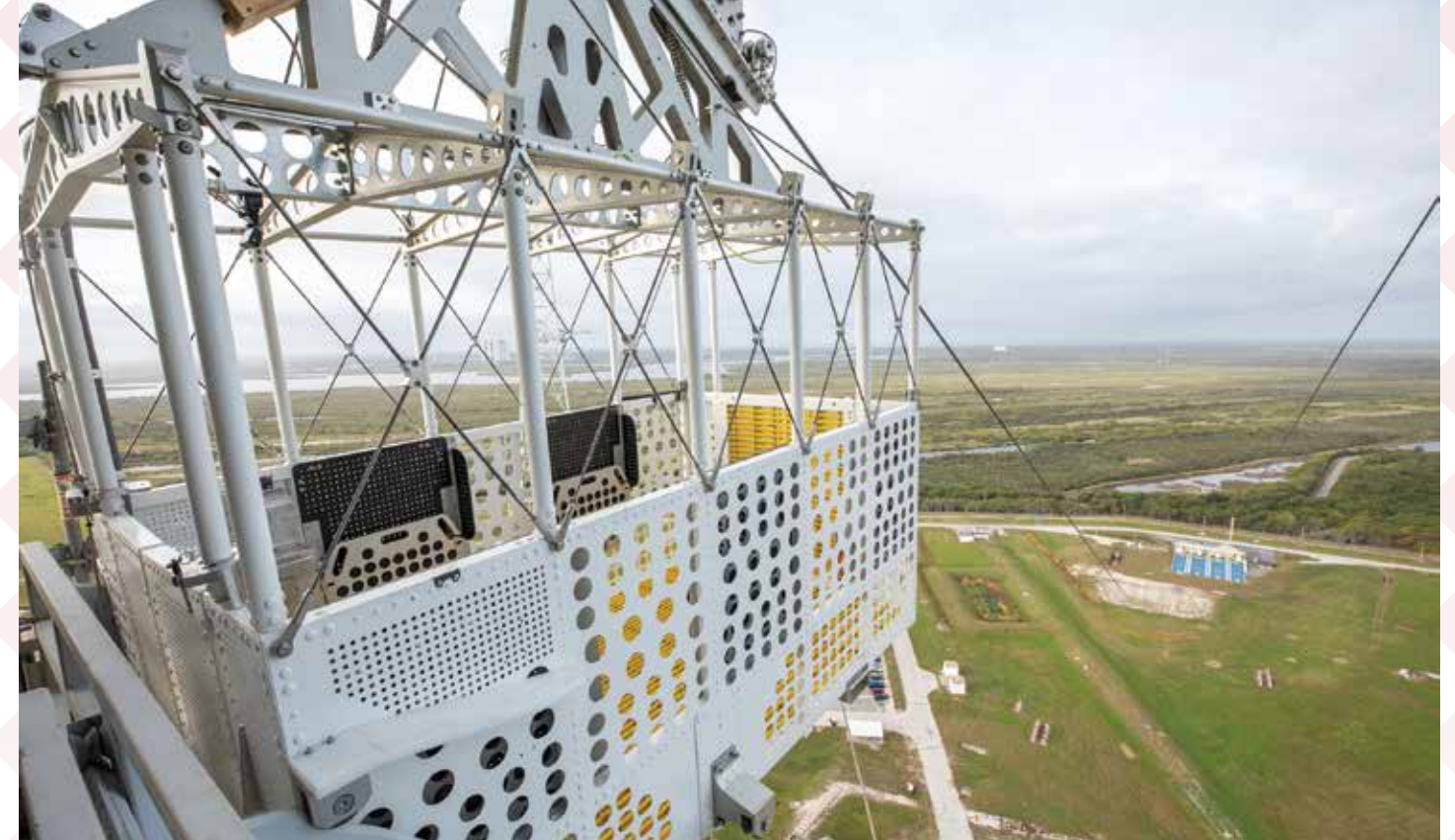
Teams with NASA's Exploration Ground Systems Program, in preparation for the agency's Artemis II crewed mission to the Moon, begin installing the first of four emergency egress baskets on the mobile launcher at Launch Complex 39B at the agency's Kennedy Space Center in Florida on Jan. 24, 2024. Photo credit: NASA/Isaac Watson
