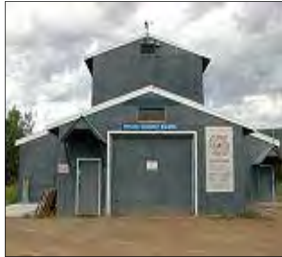
Figure 2-16. Payload Assembly Building
