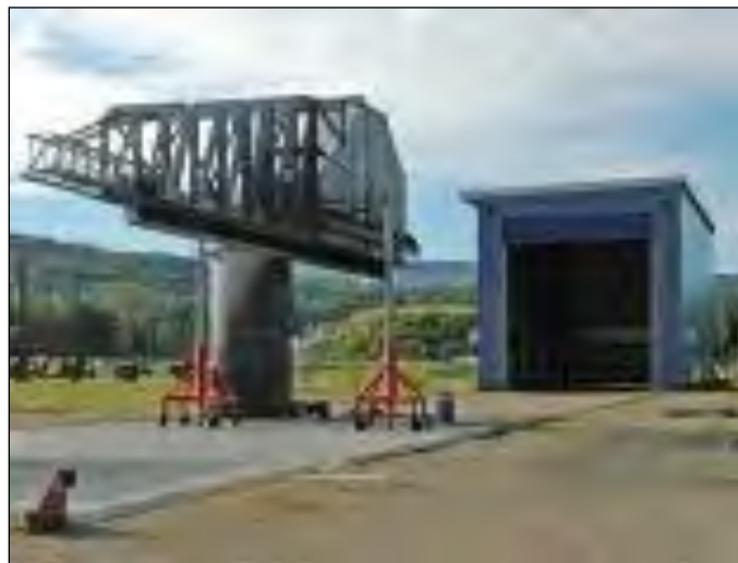
Figure 2–22. Launch Pad No. 4 with Retracted Environmental Shelter
