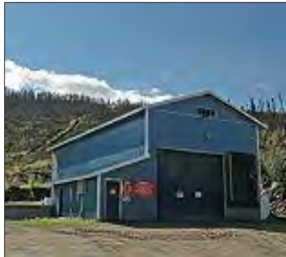
Figure 2-18. Rocket Storage Facility
