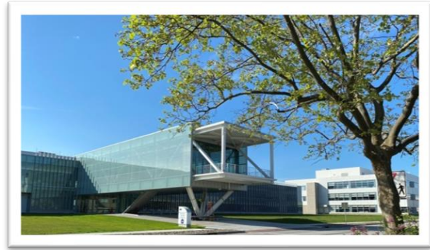
GRC Building 164, the RSB
