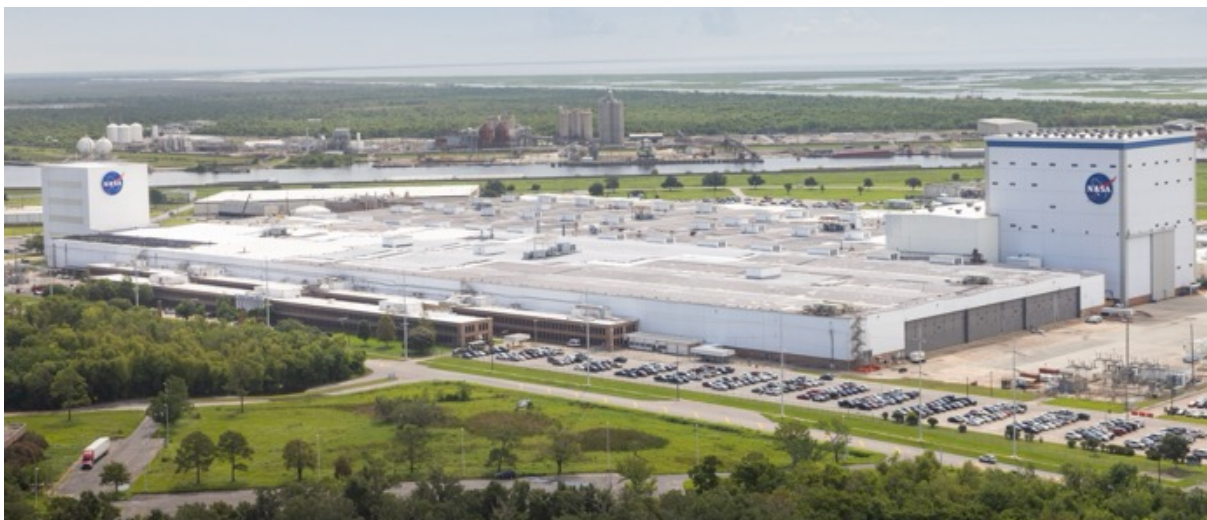
An aerial view of the main building at Michoud Assembly Facility, which features more than 43 acres of advanced manufacturing under one roof with interstate, railway and port access nearby. (NASA/MSFC/MAF)
