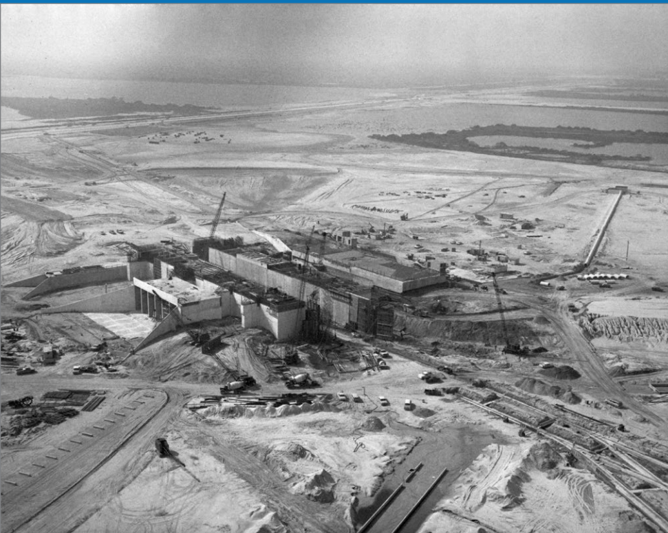
← An aerial view of early construction of Launch Pad 39A. (Photo credit: NASA)
