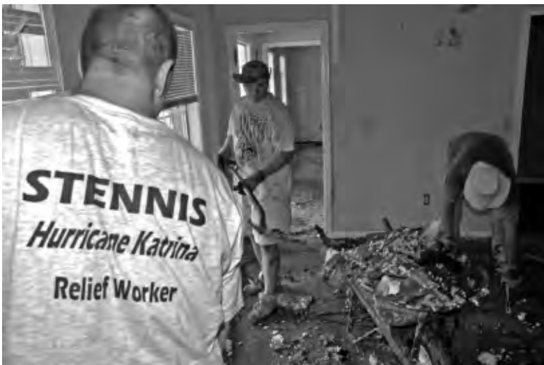
From left: Bill Graham, Troy Frisbie, and Rodney McKellip, who work at the Applied Sciences Directorate at NASA's Stennis Space Center, help tear out carpeting and dry wall from a fellow employee's house in Pass Christian on 19 September.
