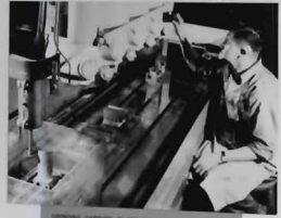
6. GRINDING THE BLADE ON GRINDWHEEL EQUIPPED WITH SPECIAL HIGH-SPEED SPINDLE
