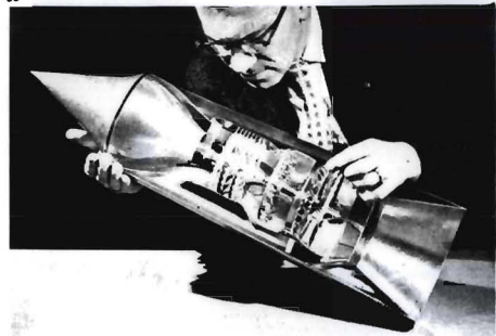
NACA scientist holds model of Mach 4 turbojet. Model has cone type variable geometry inlet, three stage compressor, very short combustion chamber and afterburner, and variable area inlet.
