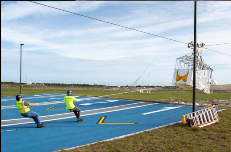
January 24, 2024—In preparation for the Artemis II crewed mission, EGS teams begin installation of four emergency egress baskets at Launch Complex 39B
