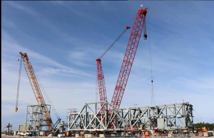
ML-2 truss work
