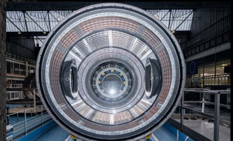
Habitation and Logistics Outpost after completion of final welds in Turin, Italy
