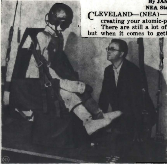
AT NACA FLIGHT LABORATORY, this dummy makes its living by going through simulated plane crashes. The seat is the latest research design to let a human survive the shock of a crash.
