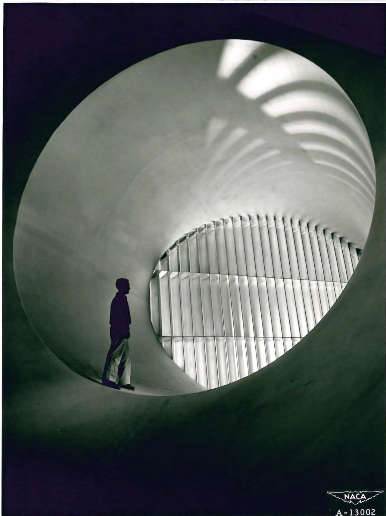
Turning vanes in the 6- by 6-foot supersonic wind tunnel.
