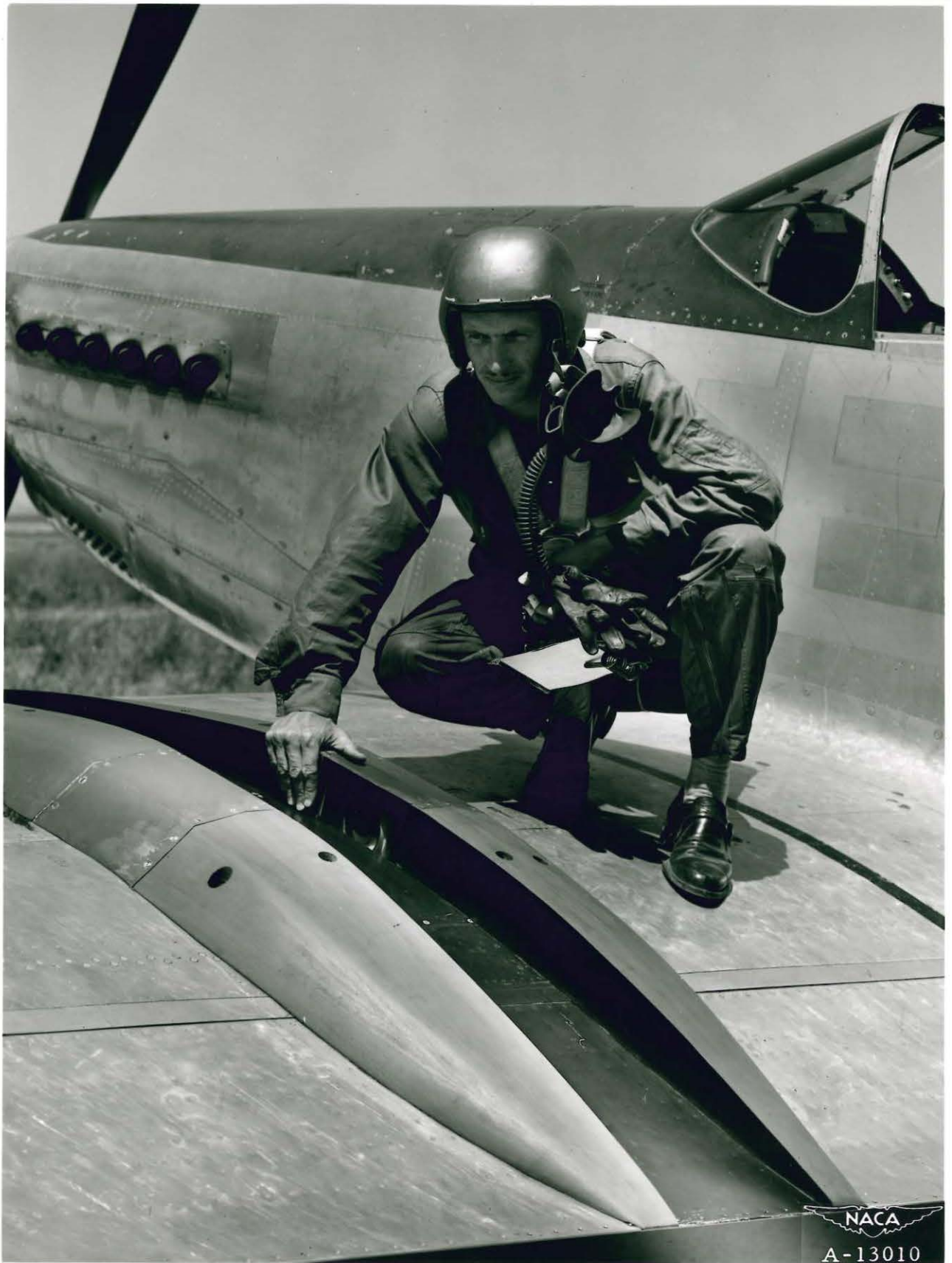
The wing-schlieren apparatus installed on the wing of a P-51 airplane.
