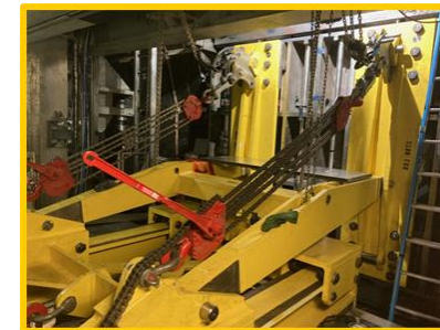
LaRC National Transonic Facility Nearside Plenum Door Repair
