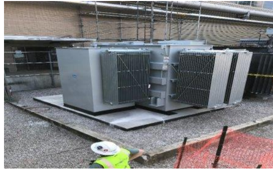
Electrical Transformer Replacement for Central Air Equipment Building
