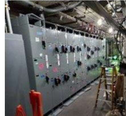
Motor Control Center Replacement for 8 Foot HTT
