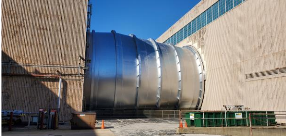
Corrosion Control of 10 x 10 Supersonic Wind Tunnel
