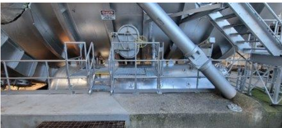
PSL Spray Receiver Tank Replacement
