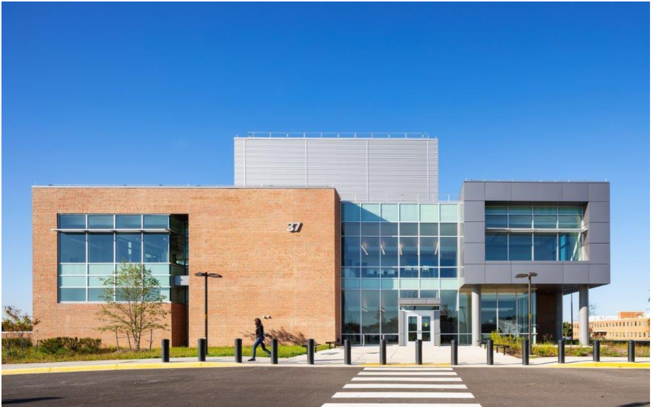
Greenbelt B37 Instrument Development Facility – 2021 Association of Builders & Contractors Excellence in Construction Award Winner
