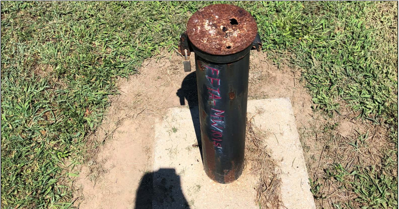
View of FFTA-MW101S and its rusted, deteriorated protective casing cover.
