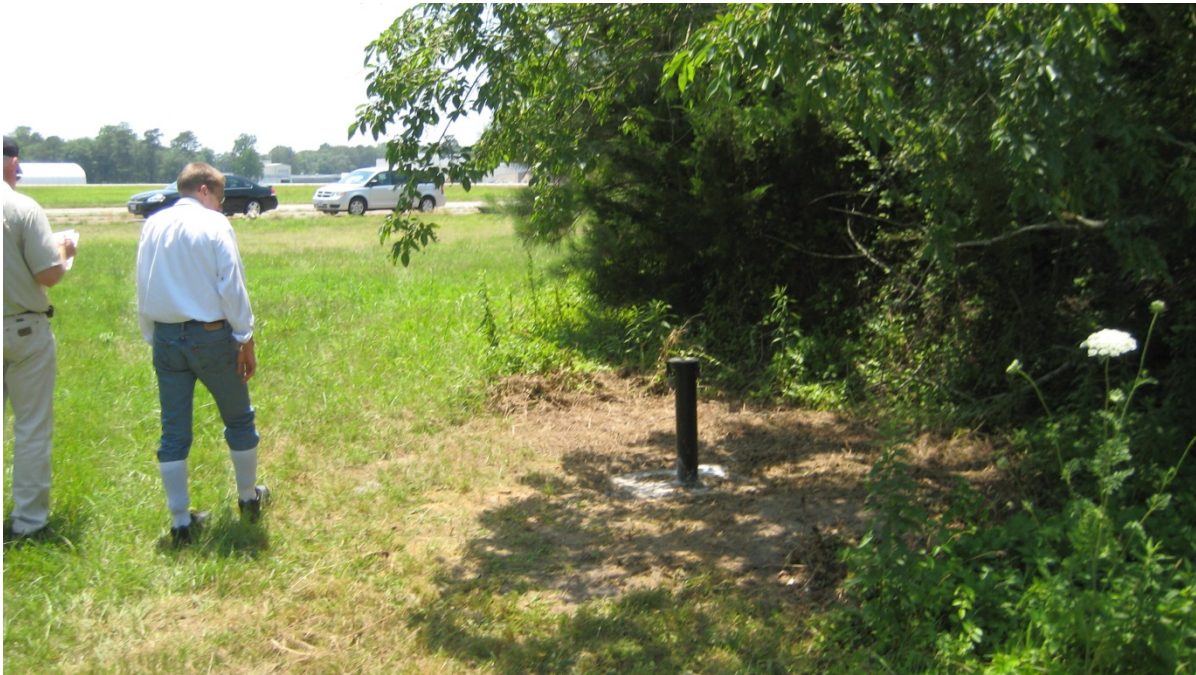
Photo 8: At FFTA-MW060I looking at the newly refurbished protective casing.
