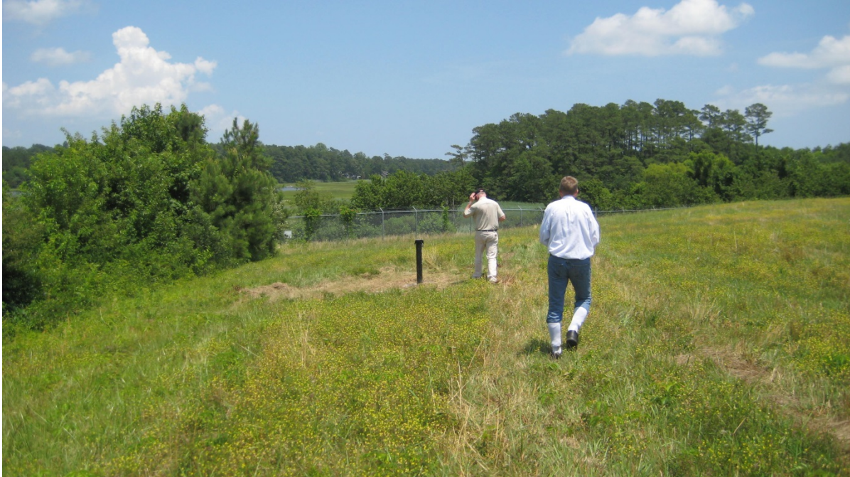
Photo 3: Looking east at WOD-MW001 which was recently refurbished.
