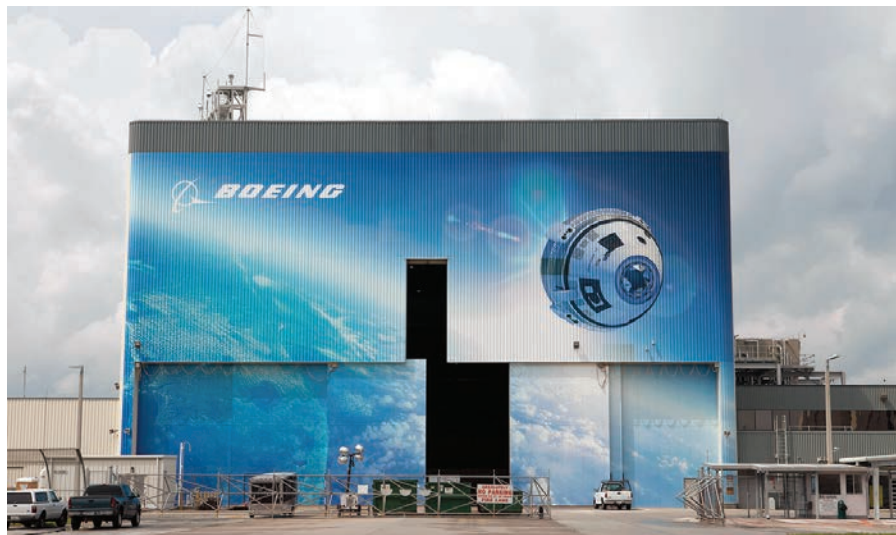
Figure 1. Boeing will be assembling and processing the Starliner at the former Orbiter Processing Facility-3, now known as the Commercial Crew and Cargo Processing Facility.
