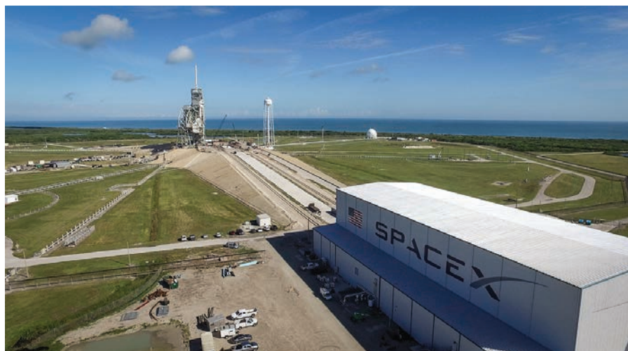
Figure 2. SpaceX has constructed a horizontal integration facility near Launch Pad 39A, planned to be used for commercial crew launches.
