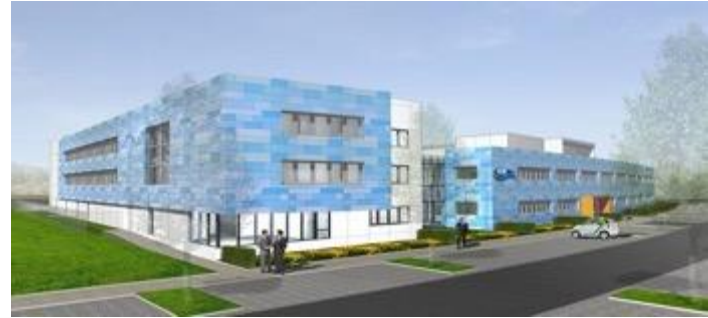
Ulm, Germany R&D Center – advanced EV battery development.
