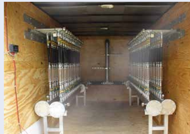
This air sparge system treats volatile organic compounds at Wilson Corners near Kennedy Parkway North and Beach Road. Photo credit: AECOM/Linnea King
