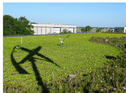
Building 12 Green Roof
