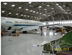
Ellington Airfield Renovated Lighting
