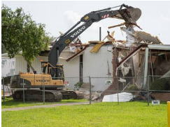
Building 226 being demolished
