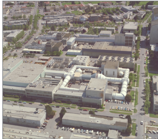
Looking west along DeFrance Avenue in 1989. From top to bottom, the 3.5-foot hypersonic tunnel, the Unitary Plan, the model shop, the 16-foot tunnel, the 7- by 10-foot tunnel, the 12-foot tunnel, and the 1- by 3-foot tunnel.
