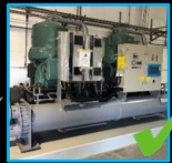
ENVIRONMENTAL CONTROL SYSTEM CHILLERS INSTALLED
