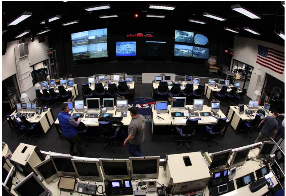
The Range Control Center before upgrade.
