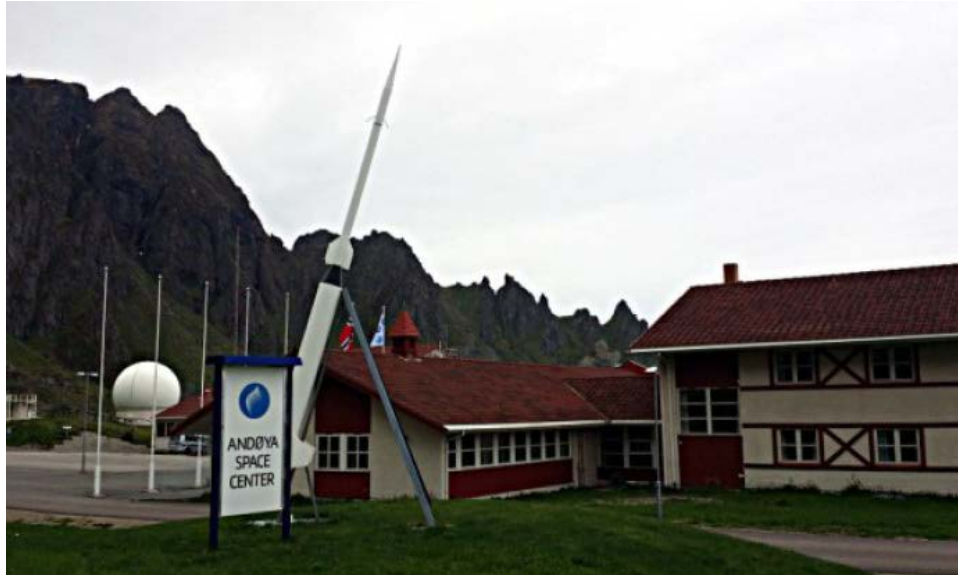
Figure B.1: Launch Facilities at Andøya Space, Photo: Kobljoern Dable
