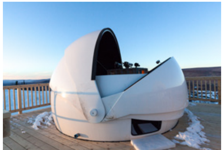
The newly installed Optical Dome located in Poker Flat Research Range.
