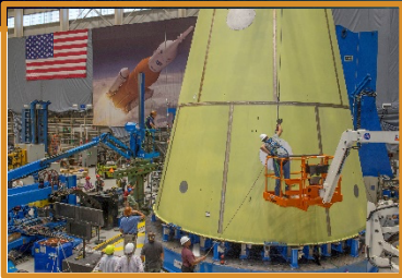
The Space Launch System Launch Vehicle Stage Adapter Manufactured in the Advanced Joining Facility
