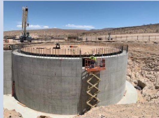
Construction of DSS-23 Antenna at Goldstone Deep Space Communications Complex
