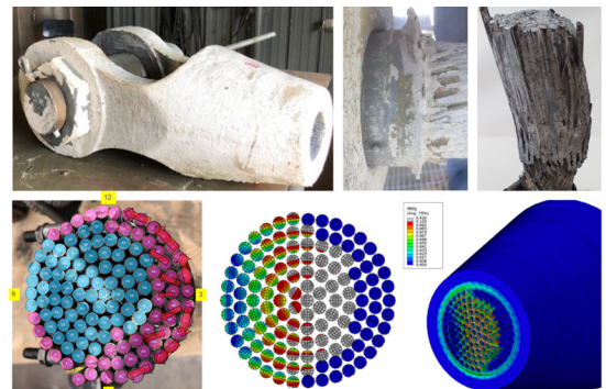
NASA Investigation of failed Arecibo Aux M4N cable/socket. Top: Socket (left); zinc extrusion (center); pulled out cable (right) Bottom: Forensic and finite element model recreation of M4N failure progression
