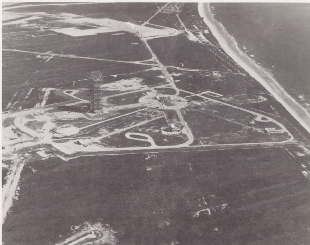
Fig. 14. LC-34 soon after its dedication. Looking north, the pad is in the center; the service structure has been removed along its parallel tracks to the parking position. The control center (blockhouse) is on the near side and left of the service structure. In the background, land is being cleared for LC-37.
