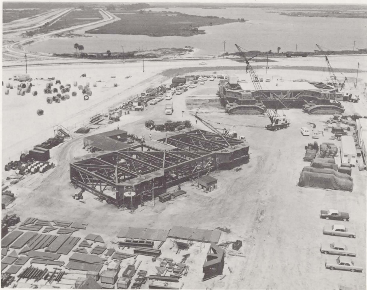
Fig. 85. Crawler-transporters under construction, April 1965.
