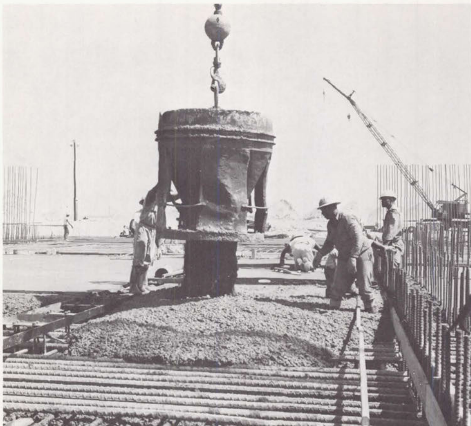
Fig. 72. Pouring the floor of the assembly building, July 1964.
