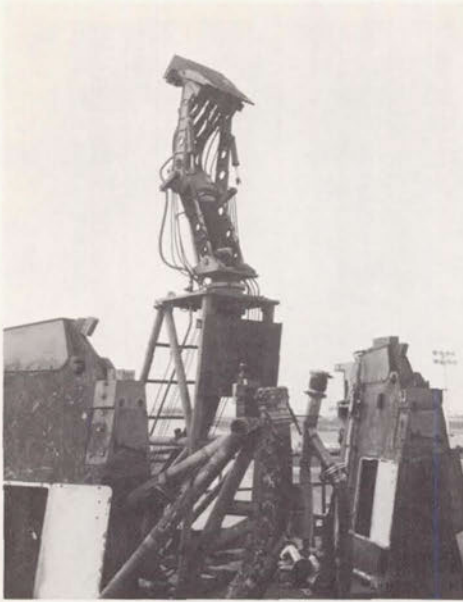
Fig. 53. Damage to pad 37B from the launch of SA-5. The short cable mast (top) carried electrical and pneumatic lines to the first stage. Access plates have been opened in the support arms (lower R and L) to inspect the pneumatic system.
