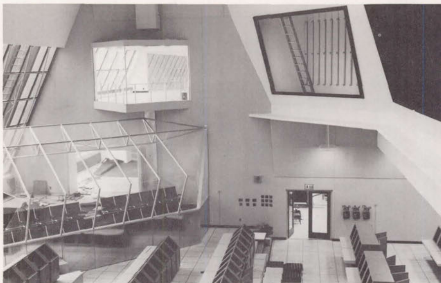
Fig. 78. Firing room 1 under construction, August 1965. The VIP viewing-area is behind the glass wall, left. The windows on the extreme left looked toward the pads. The triangular extension into the room above the VIP area was intended for the most distinguished guests.
