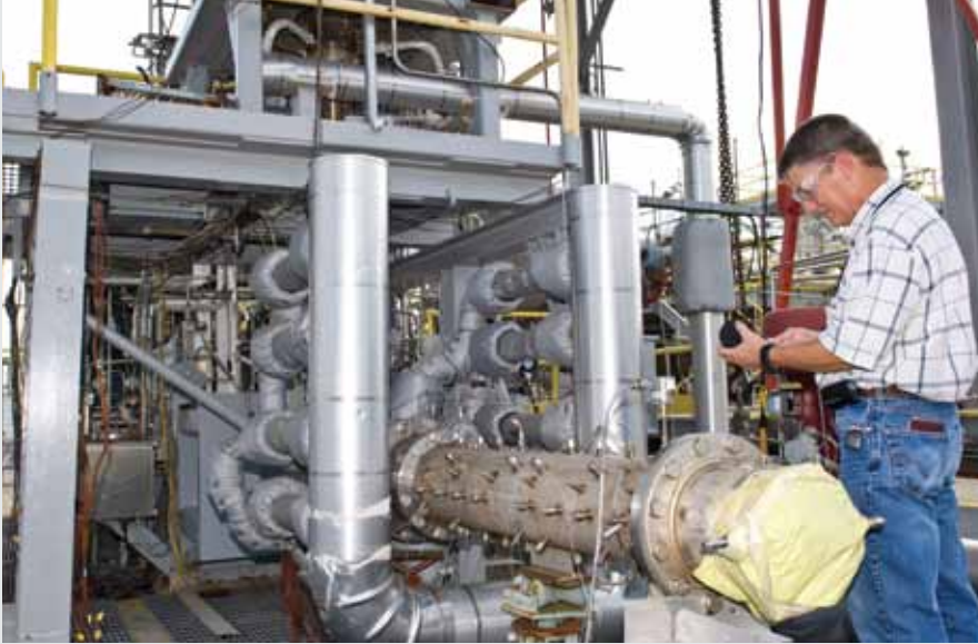
Lester Langford of Jacobs Technology, Inc. makes measurement preparations for sub-scale acoustic testing of the A-3 Test Stand.
