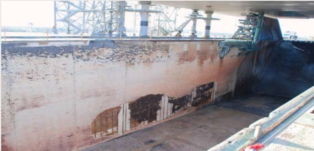
STS-124 launch resulted in over 3,000 fire bricks being stripped from the east wall of KSC Launch Pad 39-A.
