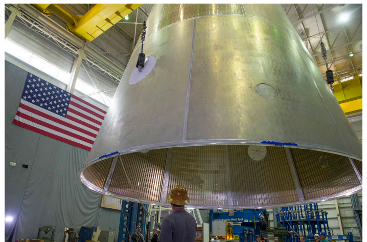
A crane lifts the qualification test article of the launch vehicle stage adapter (LVSA) after final manufacturing on a 30-foot welding tool at the Marshall Space Flight Center. The test version of the LVSA and other structural test articles for the upper part of the rocket will be tested later this year at Marshall to verify the integrity of the hardware and ensure it can withstand the forces it will experience during flight. Photo credit: NASA/MSFC/Emmett Given
