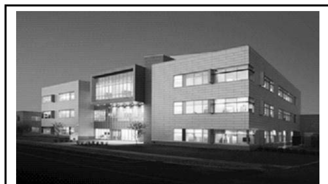
The newly constructed Mission Integration Center at GRC received Leadership in Energy and Environmental Design (LEED) Gold certification in 2014. NASA's inventory of sustainable facilities now exceeds 2.3 million square feet.
