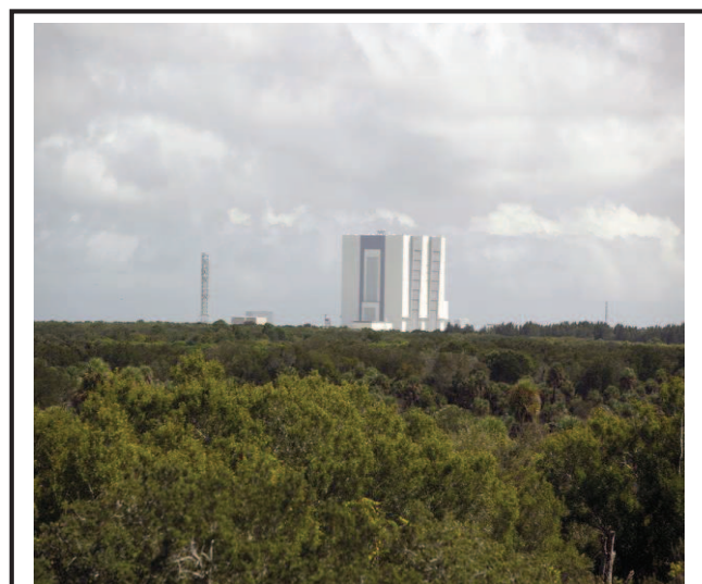
A view of the VAB at NASA's KSC in Florida. To the left is the mobile launcher that will be used to carry NASA's SLS rocket and Orion spacecraft to Launch Pad 39B for EM-1.
