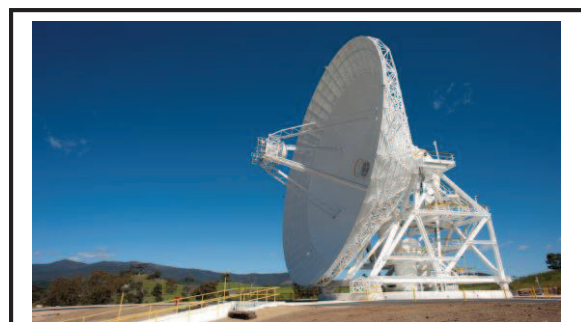
Deep Space Station - 36 (DSS-36) in Canberra, Australia, is one of four 34 meter (111 foot) Beam Waveguide antennas to be built as part of the Deep Space Network Aperture Enhancement Project. When completed, the new set of antennas will provide the same, if not higher, sensitivity and received signal power as one of the 70 meter (230 foot) antennas that have been operating for over 50 years.
