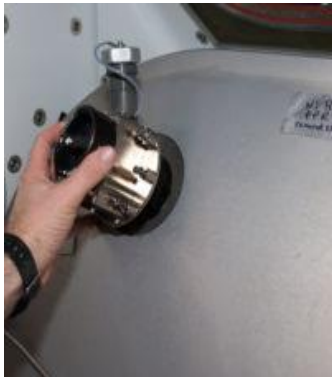
Manual Pressure Equalization Valve
