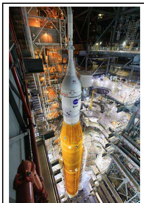
NASA's Space Launch System and Orion spacecraft atop the mobile launcher are in view in High Bay 3 of the Vehicle Assembly Building (VAB) at Kennedy Space Center. All the work platforms have been retracted in preparation for rollout to Launch Complex 39B ahead of launch of Artemis I.
