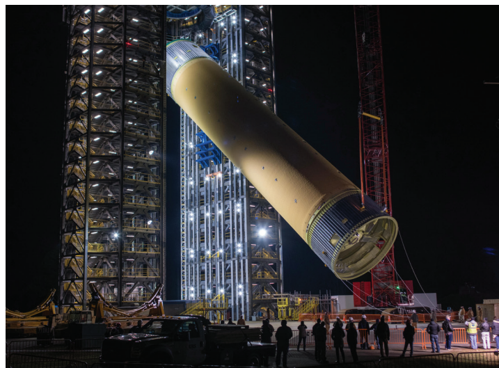
Technicians installed the liquid hydrogen tank structural test article in its test stand at Marshall at night when winds were minimal.
