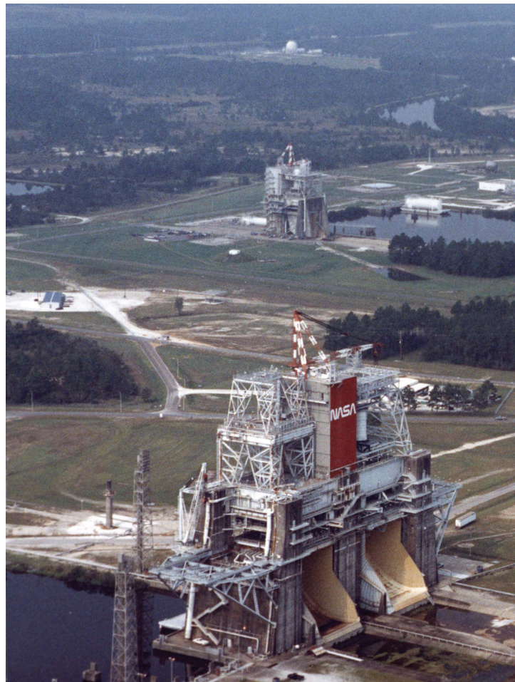
NASA Stennis provides unique facilities for testing SLS RS-25 engines and controllers. The B Complex, foreground, was used for Green Run testing the SLS core stage.
