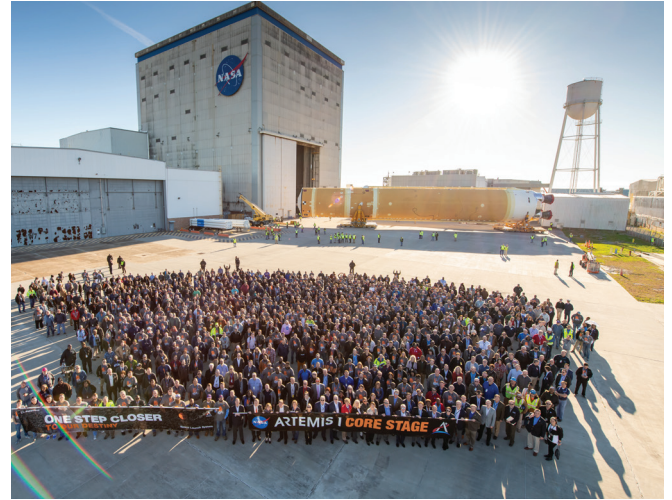
Michoud is managed by Marshall and is the world's premier rocket factory and one of the largest manufacturing facilities in the world, with 43 acres under one roof.
