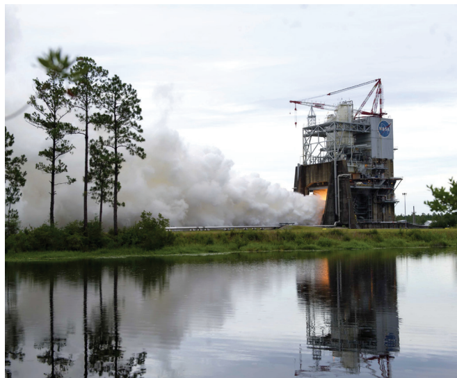
RS-25 engine and controller hot fire testing at Stennis.
