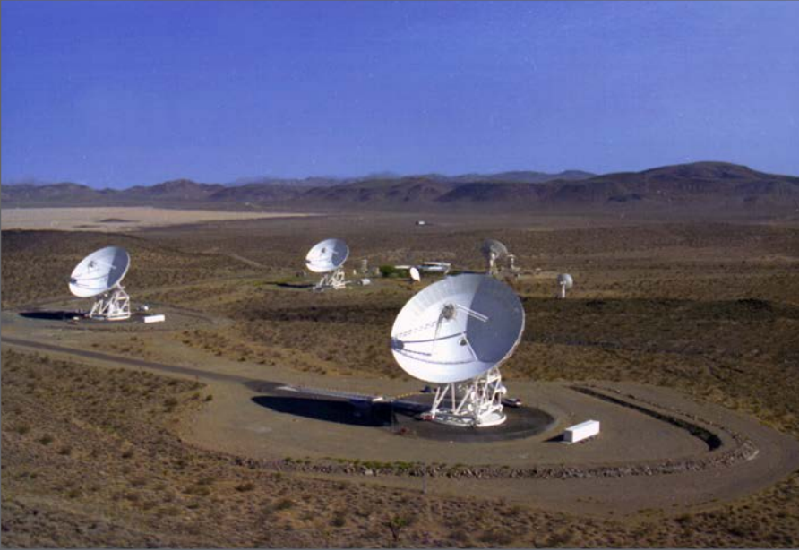
Goldstone Deep Space Communications Complex in the Mojave Desert, California. (NASA: JPL-28311)
