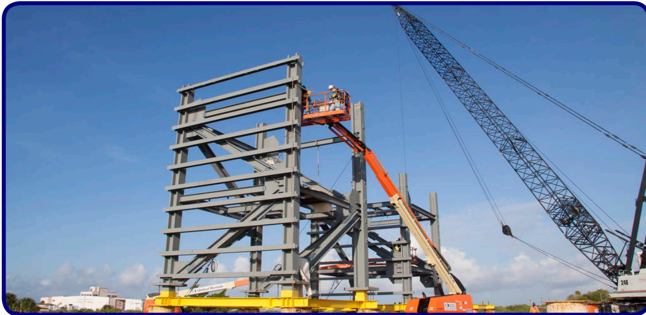
Image Caption: The first crew access tower tiers begin to take shape at Space Launch Complex-41 for flights aboard the Boeing CST-100. (Credit: NASA/Jim Grossman)
