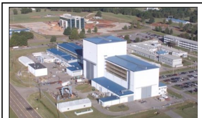
Building 4619 at Marshall Space Flight Center (MSFC) is shown above. Its mission-critical laboratories require temperature and humidity control to operate their test equipment. The building's Apollo-era HVAC system is expensive to repair, difficult to maintain, and prone to failures that impact mission test activities. The project to revitalize its mechanical systems will allow it to reliably support the laboratory testing critical to the Space Launch System (SLS), Orion, the International Space Station (ISS), and Solar Probe Plus.
