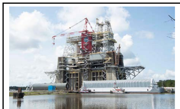
The Pegasus barge is shown here delivering Space Launch System (SLS) Core Stage Pathfinder to the B-1/B-2 test stand for practice lifts and fit checks in 2019 at Stennis Space Center in Mississippi.
