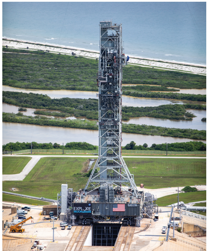
A wet flow test at Launch Pad 39B on September 13, 2019, tested the sound suppression system that will be used for launch of NASA's Space Launch System for the Artemis I mission. During the test, about 450,000 gallons of water poured onto the Pad B flame deflector, the mobile launcher flame hole and onto the launcher's blast deck. Photo credit: NASA/Kim Shiflett
