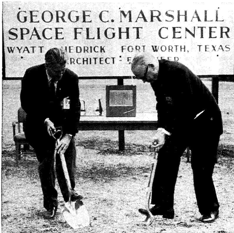
BREAK GROUND —Dr. Wernher von Braun (left), MSFC director, teams up with Sen. Robert S. Kerr, chairman of the Senate Committee on Aeronautical and Space Sciences, to break ground for MSFC's new Central Laboratory and Office Facility. The brief ground-breaking ceremony was held Saturday morning.
