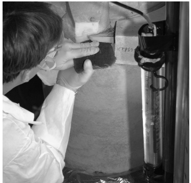
As an interim measure before the new titanium liquid oxygen (LO2) feedline bracket redesign flies on ET-128, four feedline brackets (stations 1129, 1623, 1377, and 1871) on ET-120 were modified with a different foam configuration at the Kennedy Space Center. (Photo credit: NASA/KSC)
