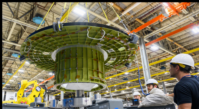
Orion crew module pressure vessel welding has begun at NASA's Michoud Assembly Facility
