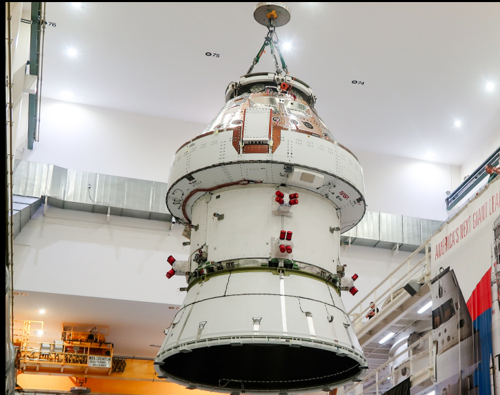
Artemis II Orion Spacecraft is lifted into an altitude chamber at NASA's Kennedy Space Center for electromagnetic interference/compatibility testing
