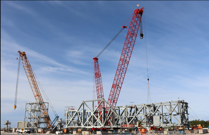
ML-2 truss work
