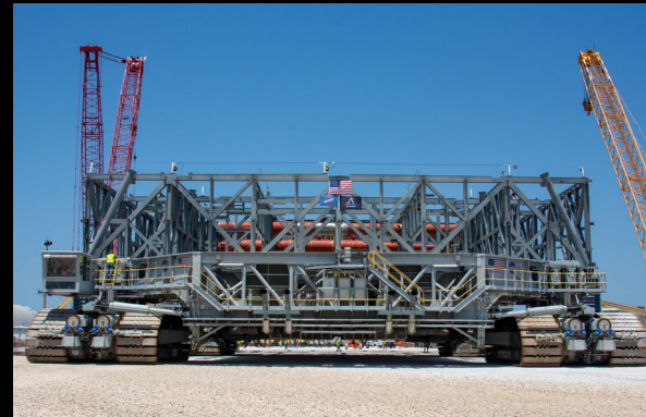
Teams with NASA's Exploration Ground Systems Program and primary contractor, Bechtel National, Inc., move the base structure of ML2 to a permanent mount structure
