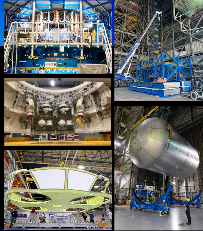
Images (L to R): 1) European Service Module (ESM) 3 undergoing final propulsion testing in Bremen, Germany; 2) KSC's Vehicle Assembly Building High Bay 2 vertical tooling progressing with first working platform installation in progress; 3) Artemis III left-hand thrust vector control buildup in work in Booster Fabrication Facility; 4) Artemis III core stage boattail lift at Michoud; 5) Artemis III LOX tank at Michoud.
