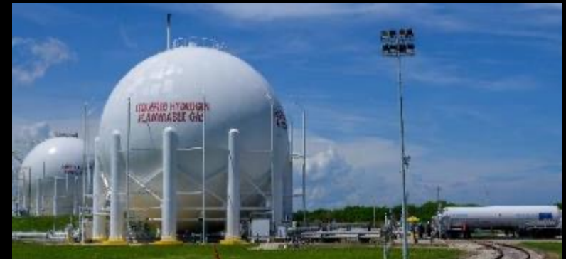
New LH2 Sphere at the Pad for Artemis II
