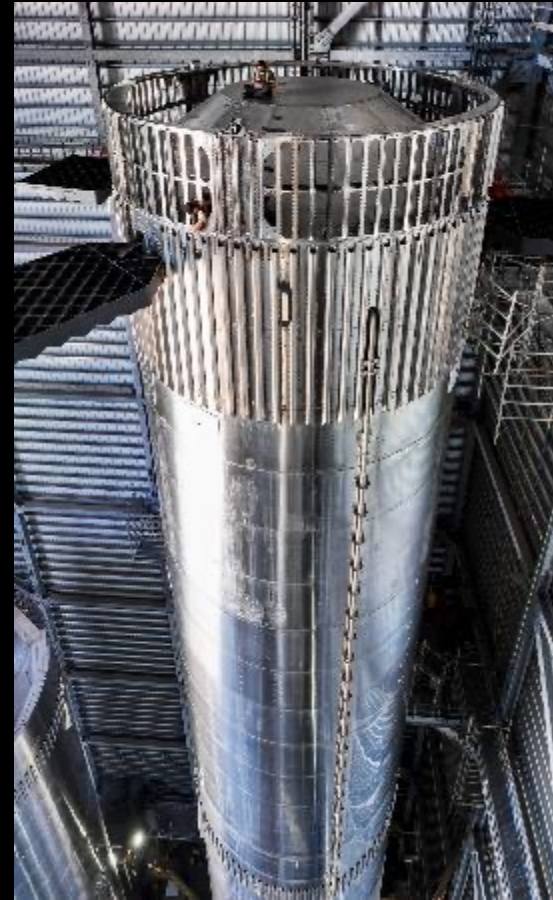
Aug 18, 2023 - Vented interstage and heat shield installed atop Super Heavy Booster 9, an upgrade for a new separation method called hot staging, where Starship's second stage engines will ignite to push the Starship away from the Super Heavy Booster.
