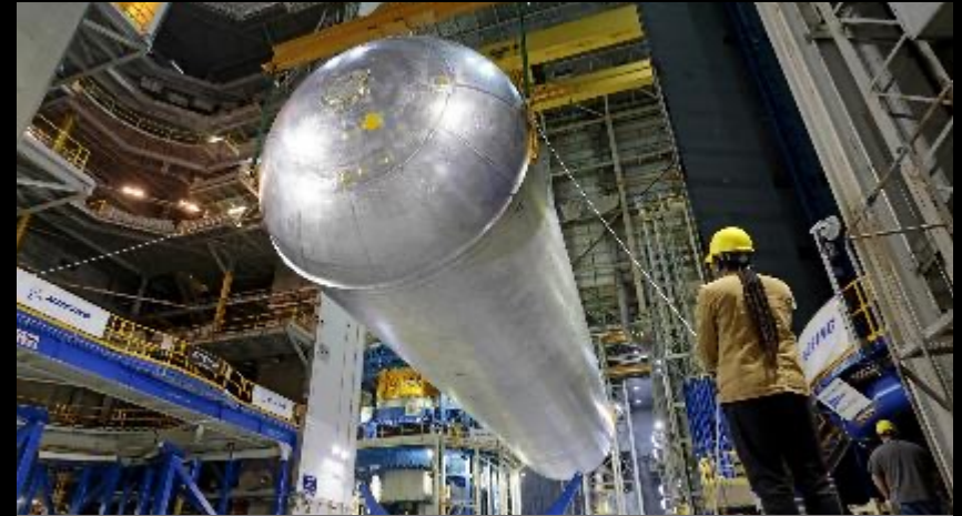
Artemis III Space Launch System Core Stage Liquid Hydrogen Tank
