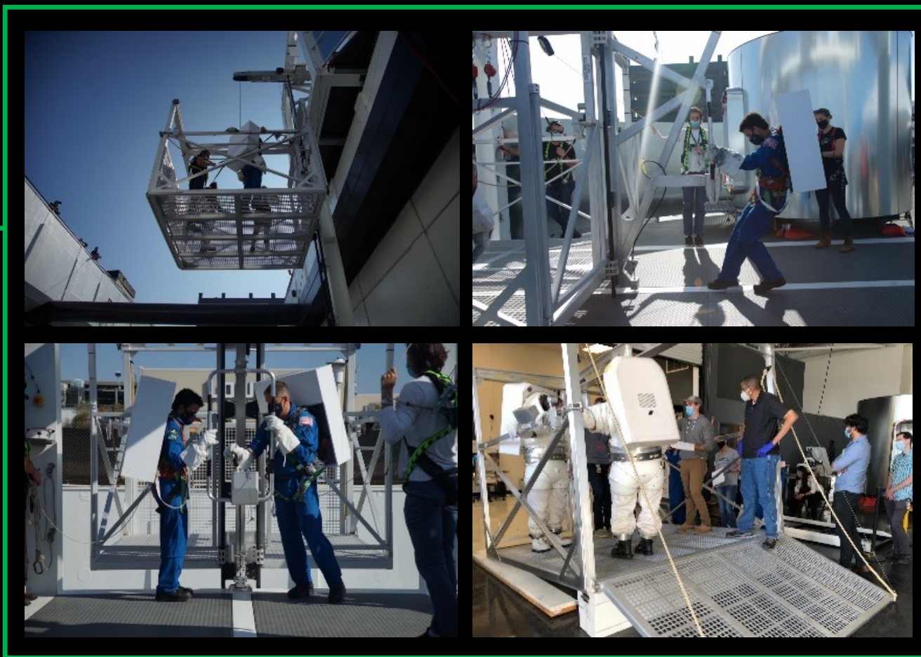
Crew and Cargo Elevator
