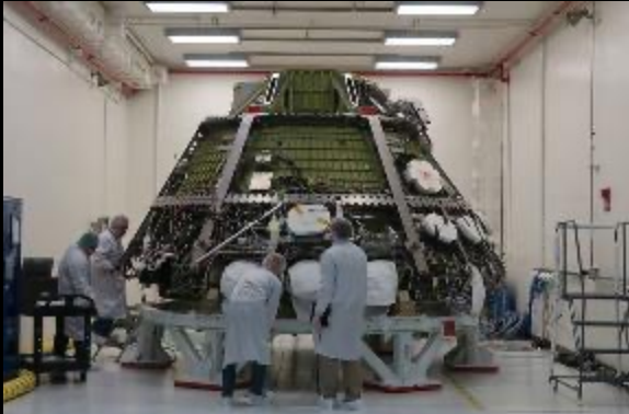
Crew Module ECLSS Bay Components Installed
